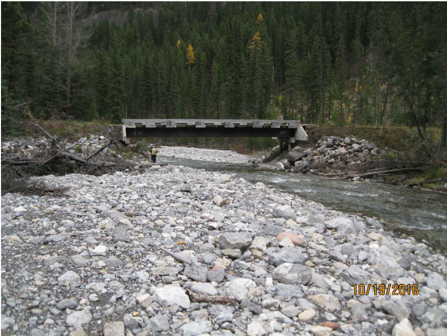
4 10 PHOTO 4 - EXISTING BRIDGE FROM UPSTREAM SCALE: NTS
