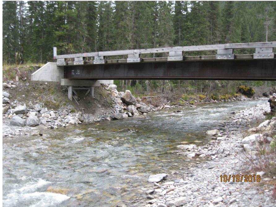
5 10 PHOTO 5 - EXISTING BRIDGE FROM DOWNSTREAM SCALE: NTS
