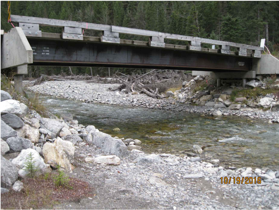
1 10 PHOTO 1 - SITE OVERVIEW SCALE: NTS
